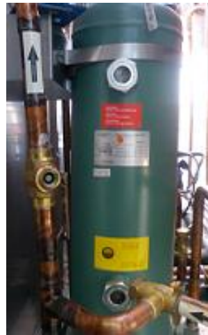
Air Dryer in Condenser Unit
