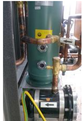
Air Dryer in Condenser Unit
