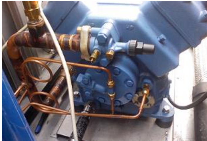
Compressor for Central HVAC system
