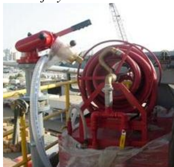
Firefighting system for Helideck
