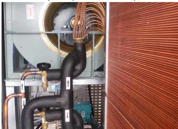
Air Handling Unit (AHU) for Central HVAC system
