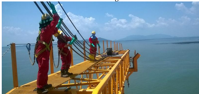
Lurication for wire rope after Load test of Crane
